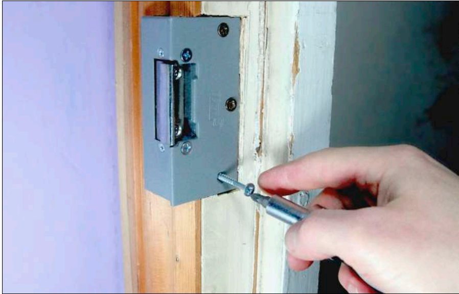
Figure 8-13: Installing the door strike.
